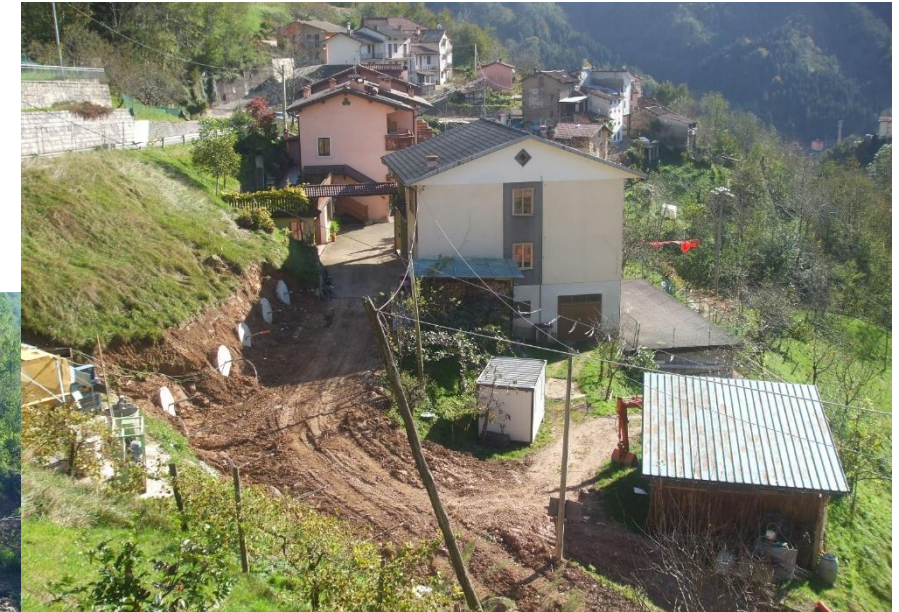
Cischele landslide (Recoaro Terme, VI)
